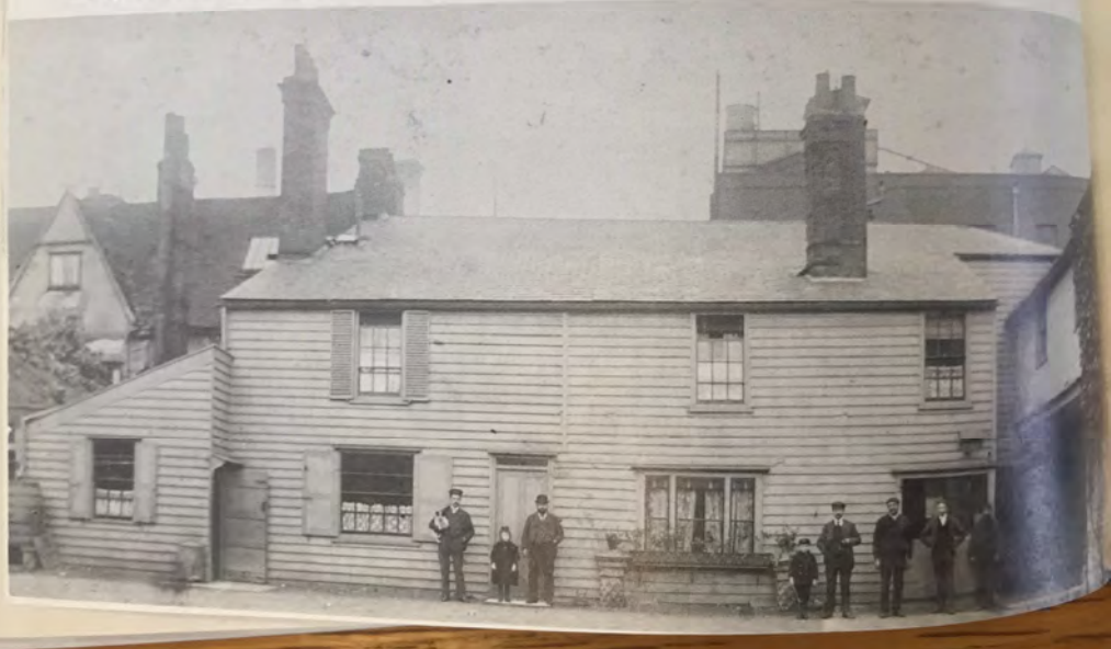
101. A rare glimpse of backyard Romford in 1895. The less public side of the Coach and Bell is a neatly-kept house. On the top of the roof, to the right, the brewery frontage can be seen.
