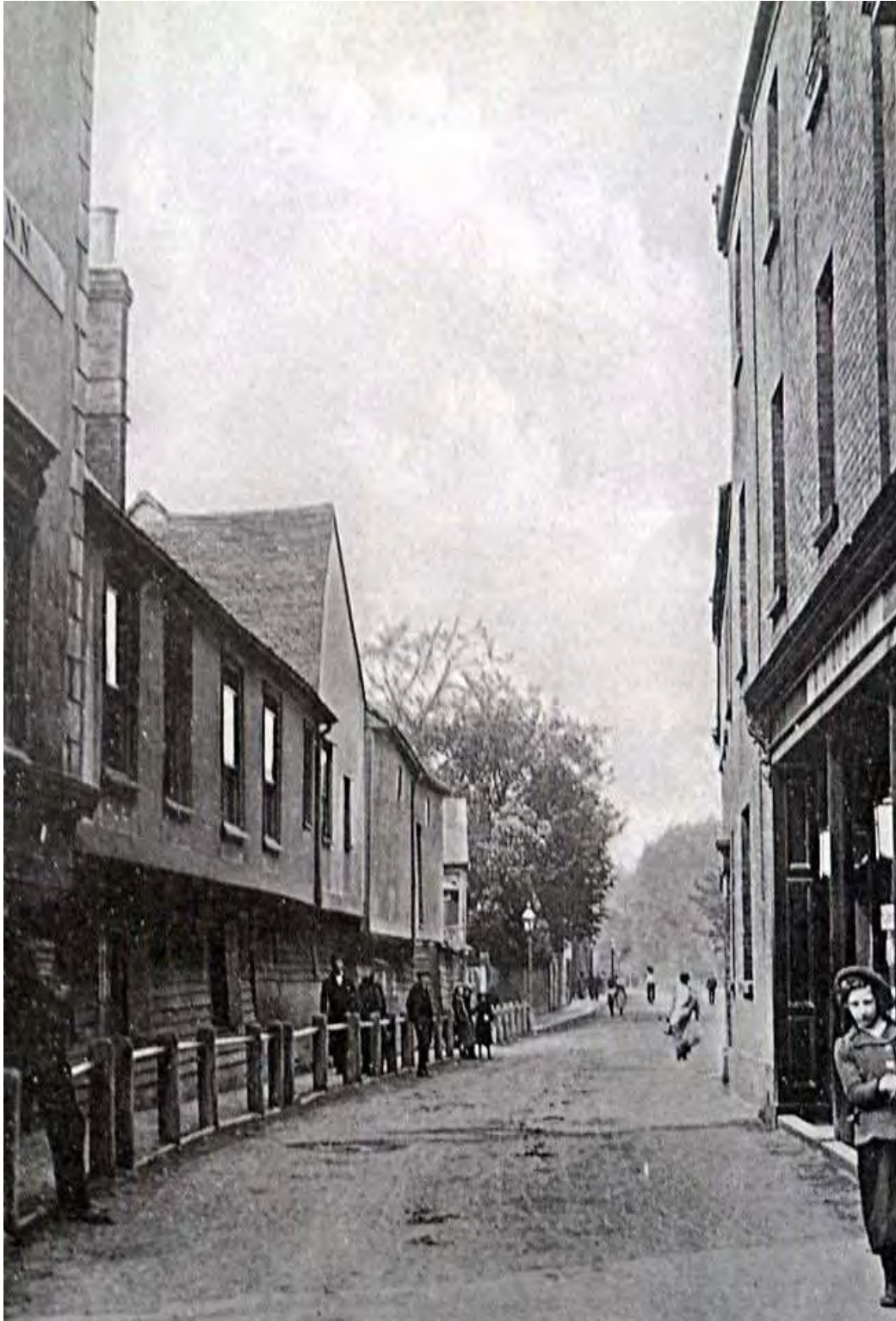
North Street with a glimpse of the vicarage garden beyond the flank of the Golden Lion and further trees closing the vista.
