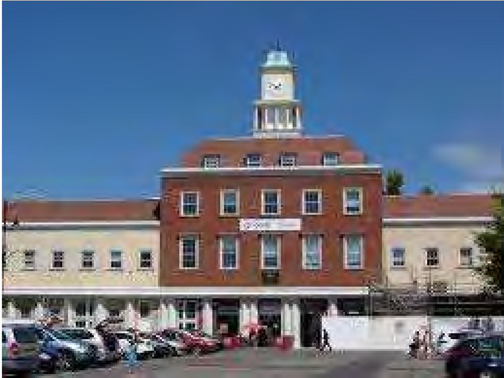
The pastiche Tollgate House, completed c.2013 to close the east end of the market in a manner akin to the prior Laurie Hall.
